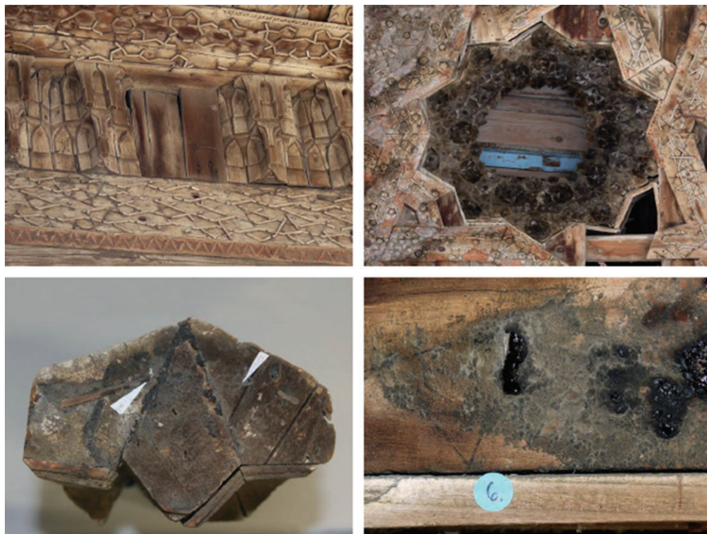
Figure 1 Detail of the Khoja Zaynuddin Mosque: (a) the ceiling of the portico, with cornice muqarnas; (b) the ceiling of the portico, with central muqarnas; (c) a section of the portico muqarnas showing the presence of glue; (d) a close-up image of the glue used to construct the portico.
